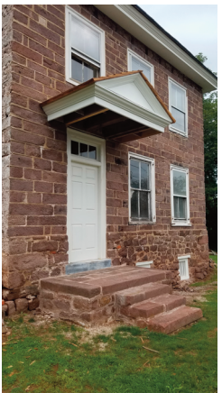
Restored front door with marble threshold and triangular hood
