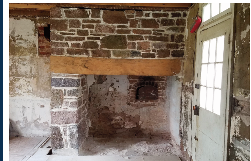
Restored kitchen hearth built of local red sandstone and a hand-hewn oak lintel
