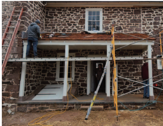
Side porch restoration in progress
