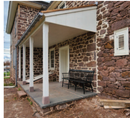
Side porch restoration after completion
