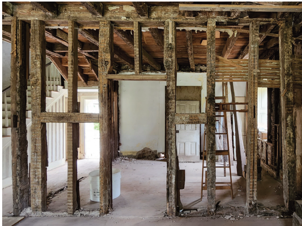
First-floor wall partition constructed in German Fachwerk or "half-timber" framing. An original door opening is in the middle, leading from the front room to the kitchen.
