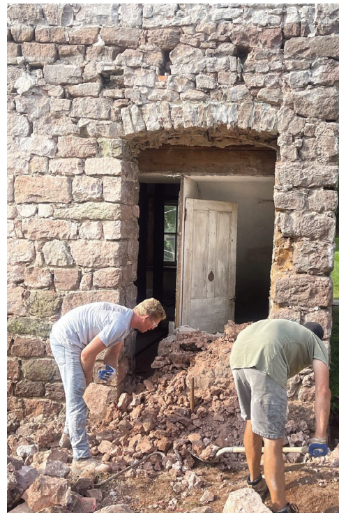
The original masonry arch above the rear door opening was exposed during stucco removal.
